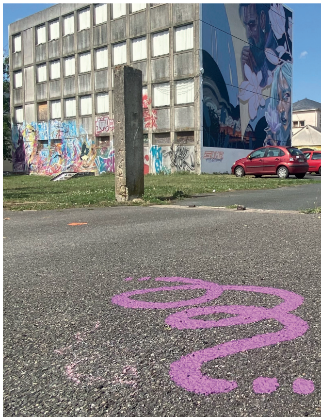
Metro Europa line in Bourges northern outskirts
