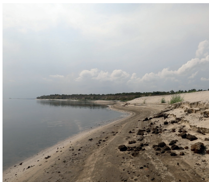
Zaporizhia, Dniepr river after destroyed dam © Opera del Mondo
